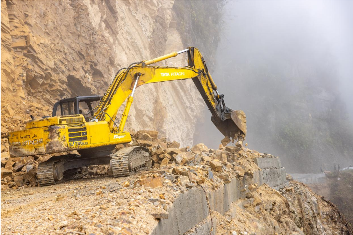
Heavy excavator performing road construction and rock clearance, Aalo, Arunachal Pradesh
