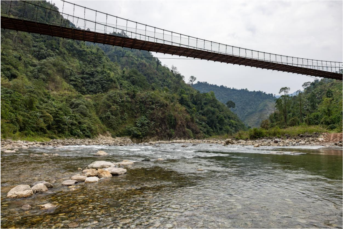
Suspension Bridge Spanning Yamne River, Katan, Arunachal Pradesh
